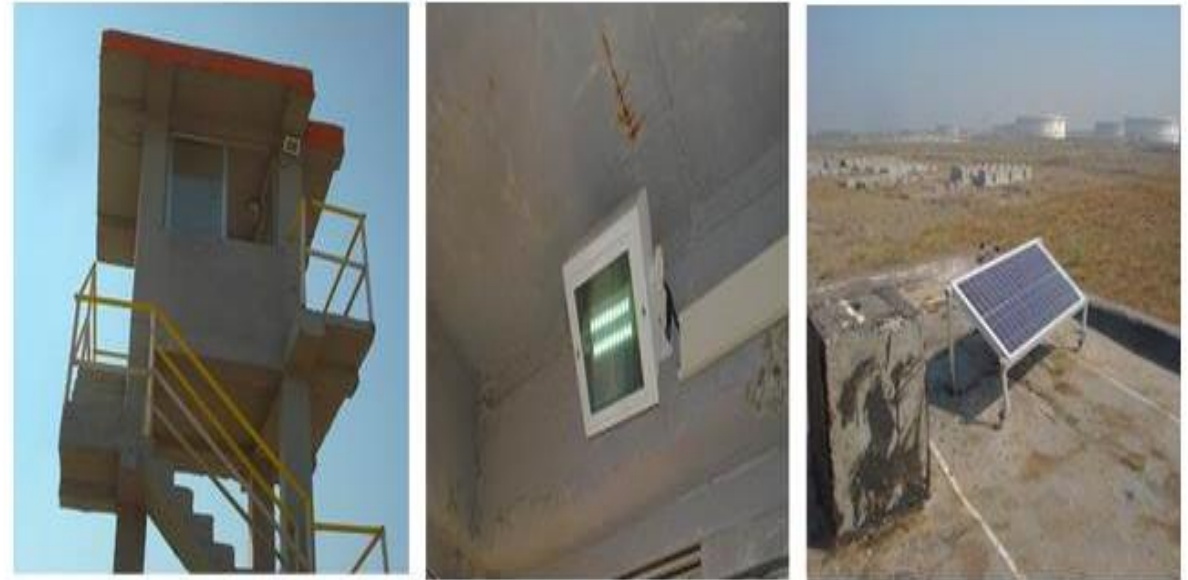
Boundary Security watch towers provided with Solar Panel for lighting of Tower
